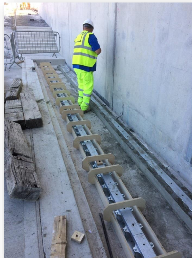
Installation of the Door Running Track
