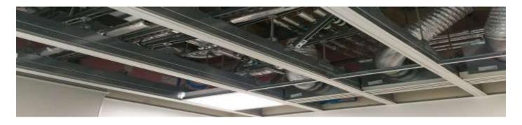
The modern hospital ward, treatment room or imaging room is a crowded environment and much equipment needs to be suspended from the ceiling capable of withstanding high static and dynamic loads. This ranges from light weight pendant lights to extremely heavy Fluoroscopy, X-Ray and Ultra sound imaging equipment which need to move quickly, smoothly and safely.
