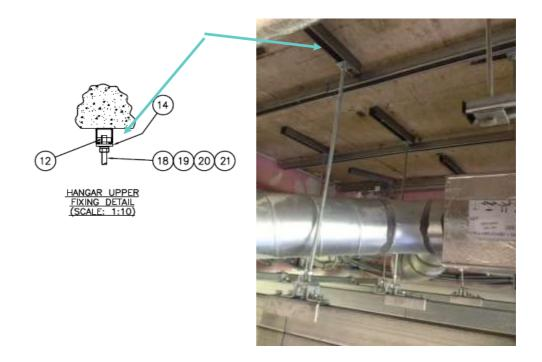
Phase 2: Secondary main P5500 Unistrut channel fitted to primary using threaded drop rods.
