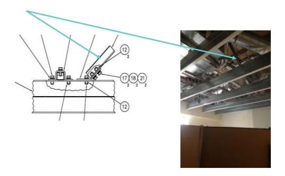
Phase 4: Ceiling tile support angle installed and tiles fitted.
